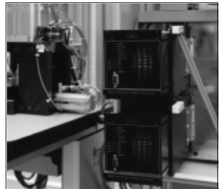
JVL AMC11B AC Servo Controllers mounted in the control cabinet.
